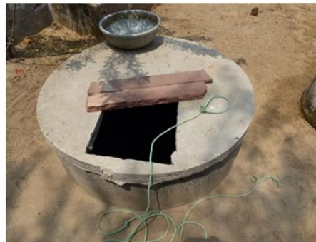
Rainwater Harvesting System
